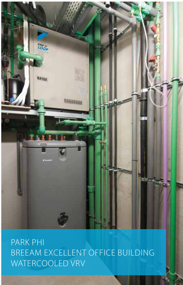
LOOP BY DAIKIN VRV IV+ HEAT RECOVERY
